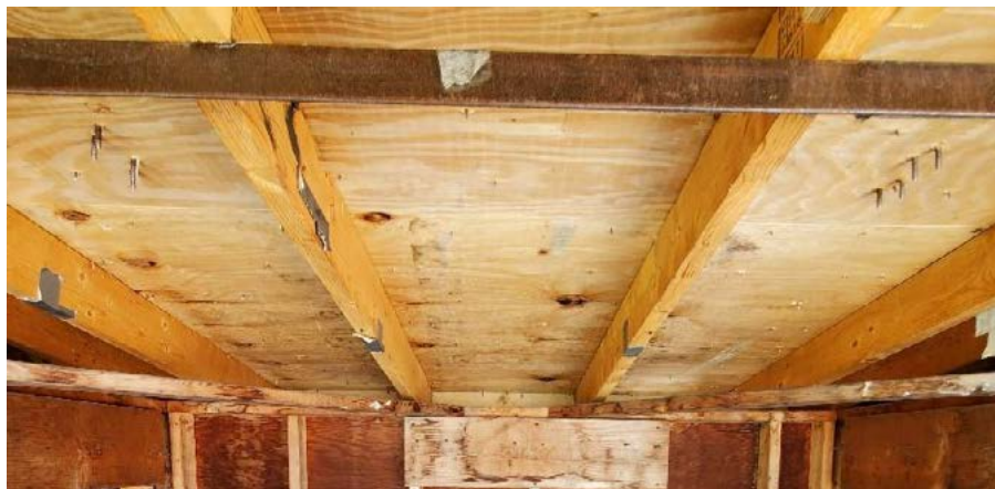
Photo No. 2 Underside Before Testing
