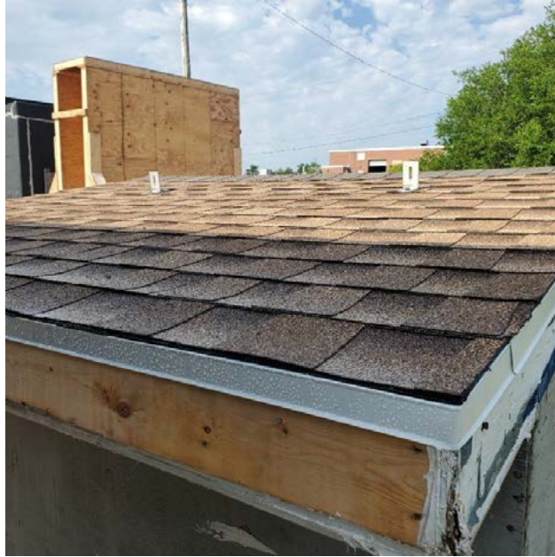
Photo No. 1 Top Side Before Testing
